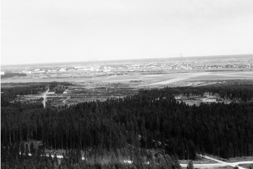
Fig. 1. Pinomäki hill stands out in the photograph from the 1950s as a tree-less clearing in the middle of the forest (visible on the right side of the image). Several German-built barracks can still be seen in the photo. On the left side of the image is the former German technical area, where a single German aircraft hangar from the war period remains. Source: Finnish Defence Forces' Photograph Archive.
